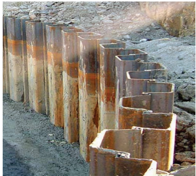
Steel Retaining Wall
