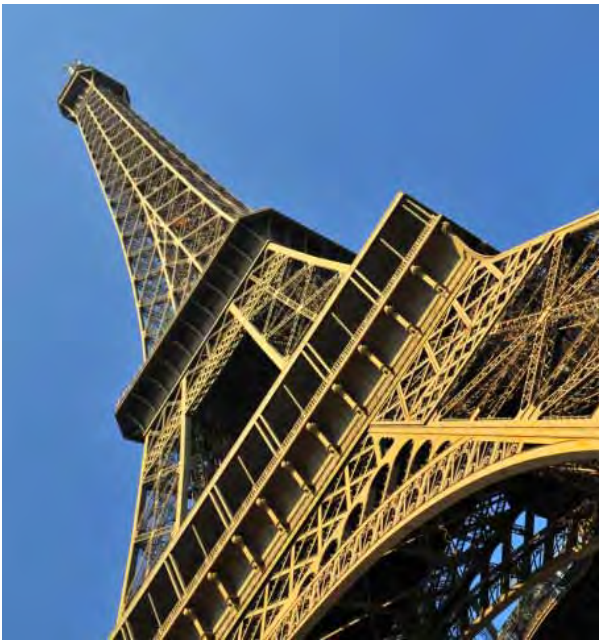
The Eiffel Tower in Paris, France: Gustave Eiffel's iconic iron lattice masterpiece contains 18,038 pieces of puddle iron and 2.5 million rivets
