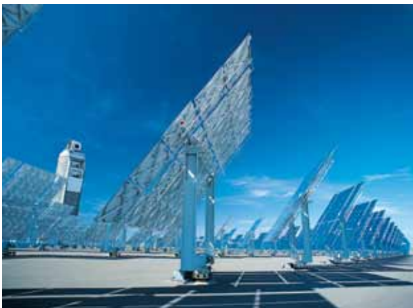
Solar power panels, Albuquerque, New Mexico, US. Steel bases are used to ensure the panels' strength and security
