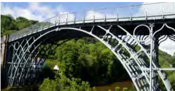
The Iron Bridge in Shropshire, England. The first arch bridge in the world to be made of cast iron - it was opened in 1781, and stands to this day
