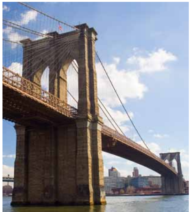
Brooklyn bridge, New York, USA (1883). This was the longest suspension bridge in the world until 1903, and the first steel-wire suspension bridge
